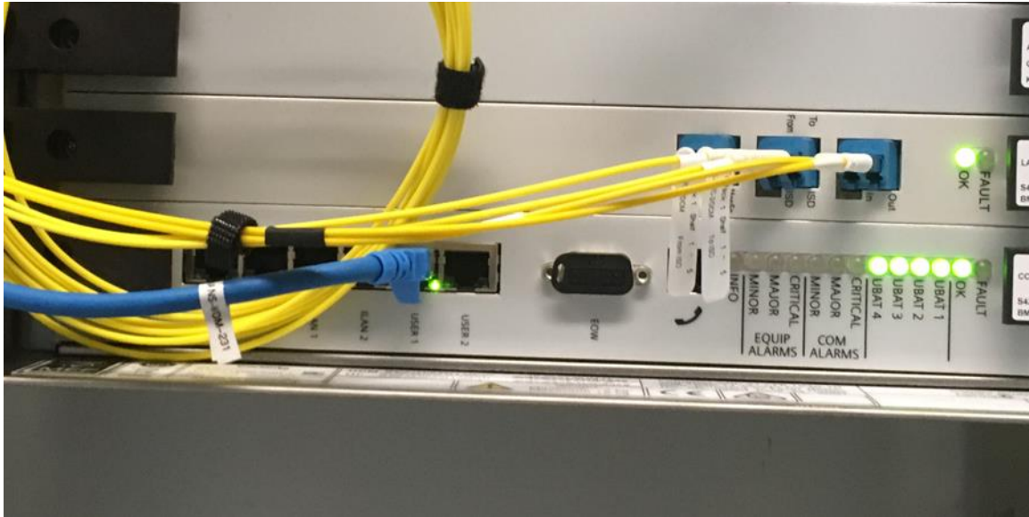
Figure 4.2: Bringing connectivity into huts to monitor metrology amplifiers through USER 1 User Port 1 (blue Ethernet cable in the picture)
