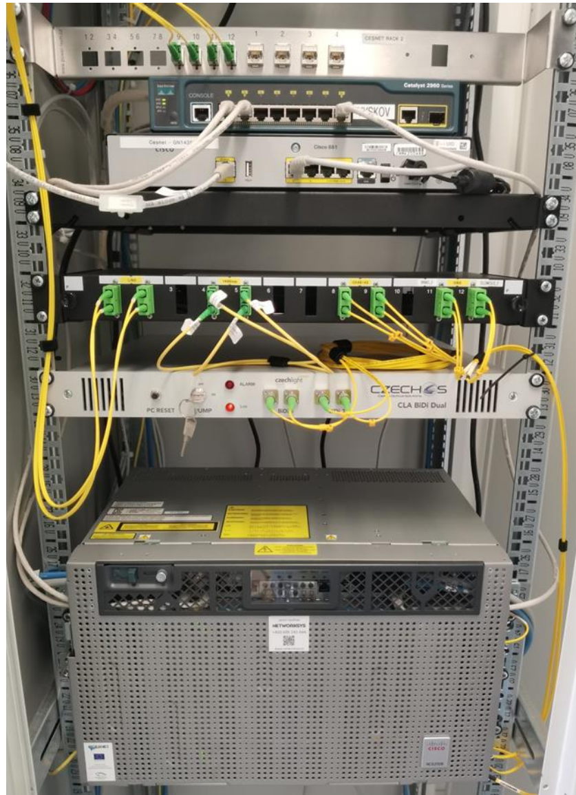
Figure 5.3: Physical view of OADM filter for multi-band S (1451 nm), C band (ch. 43–46) and L band (ch. 7)
