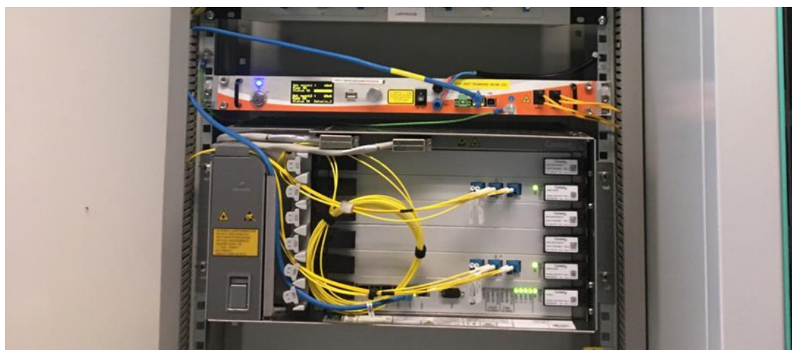
Figure 4.1: Housing of bi-directional amplifiers in ILAs
